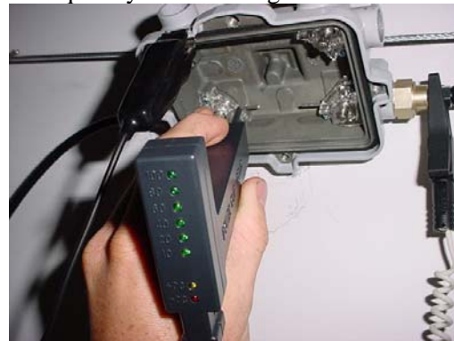
Fig 1b: Power Clip™ inside power inserter.
